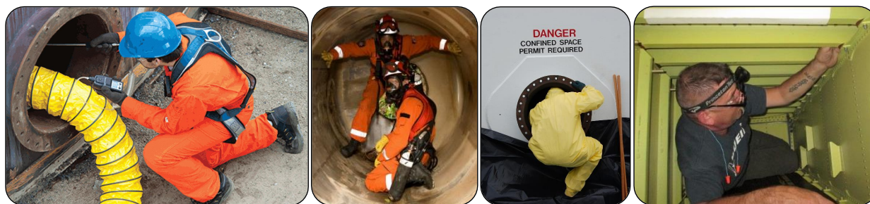
Figure 1: Examples of workers operating in confined spaces, which require unergonomic postures and present environmental hazards for workers.
